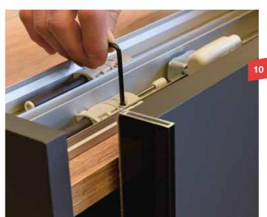
Simply practical: The door overlay can be continuously adjusted. The cabinet is finished!
