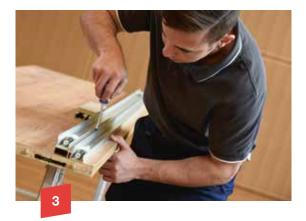
Know how: The master easily mounts the prepared guide track.
